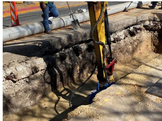
Sewer bursting pits being backfilled on 2100 South near 1200 East
